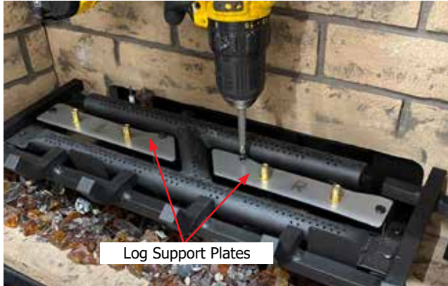
Diagram 5-Install Log support plate installation
