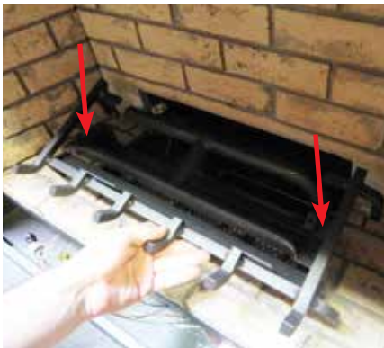
Diagram 1: Remove left and right screws.
