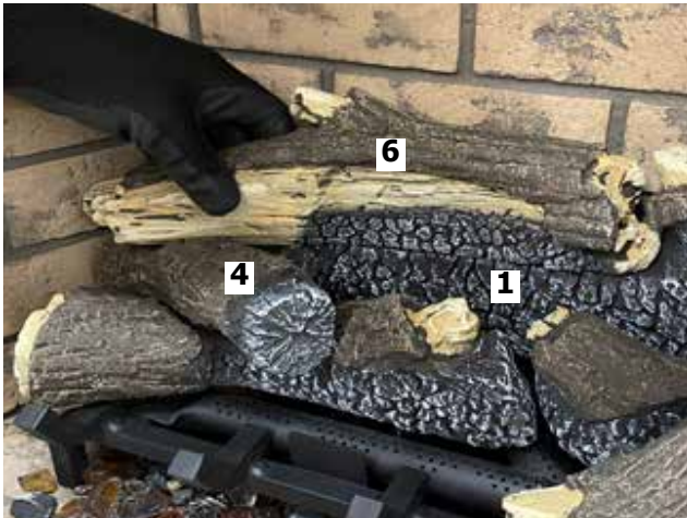
Diagram 11-Install Log 6
