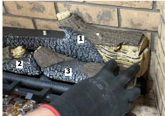
Diagram 8-Install Log 3
