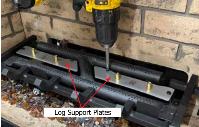
Diagram 5-Install Log support plate installation
