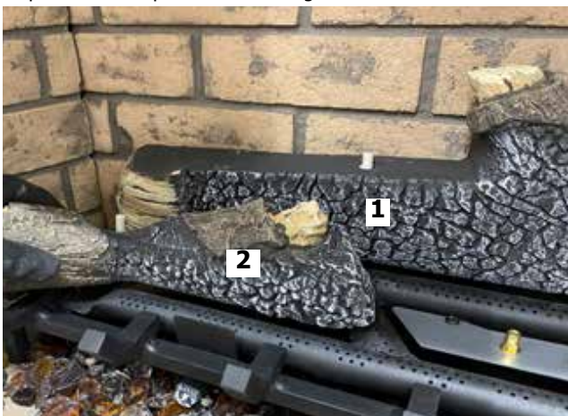
Diagram 7-Install Log 2
