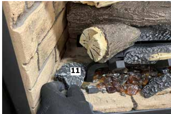
Diagram 16-Install Log 11
