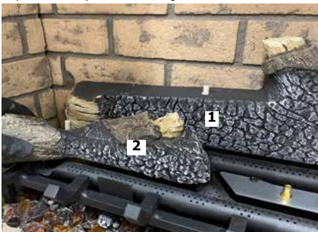
Diagram 7-Install Log 2
