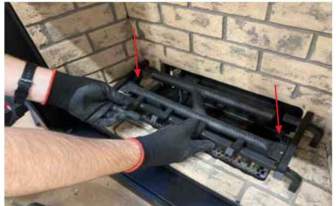
Diagram 2-Log Grate Install
