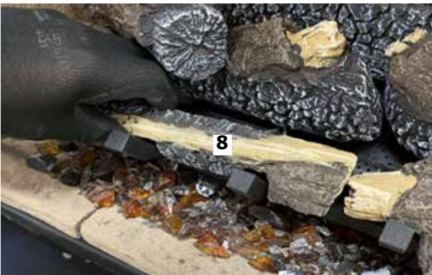
Diagram 13-Install Log 8
