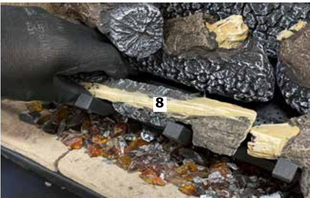
Diagram 13-Install Log 8
