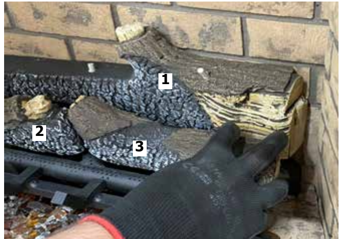
Diagram 8-Install Log 3
