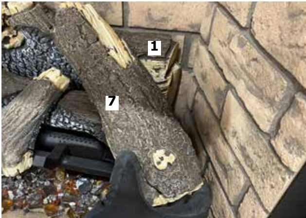
Diagram 12-Install Log 7
