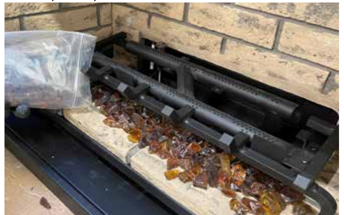
Diagram 3-Install Glass
