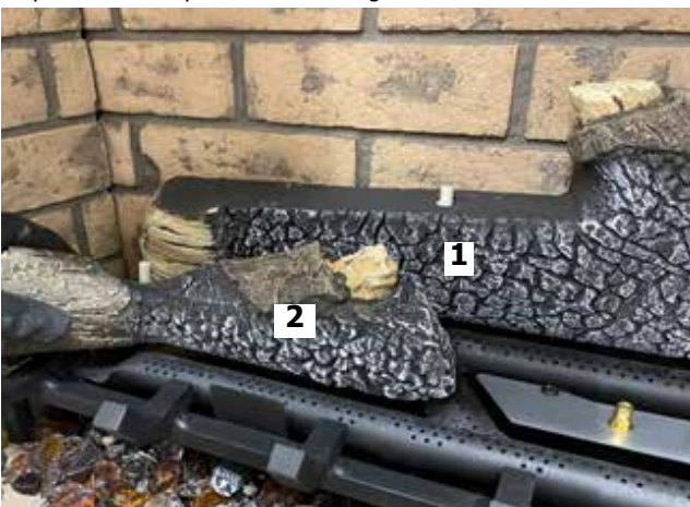
Diagram 7-Install Log 2
