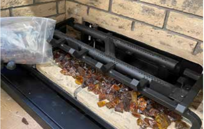
Diagram 3-Install Glass
