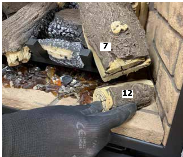
Diagram 17-Install Log 12
