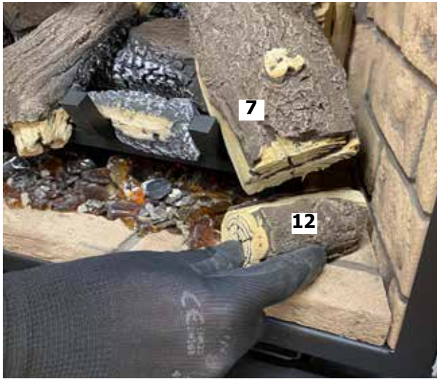
Diagram 17-Install Log 12
