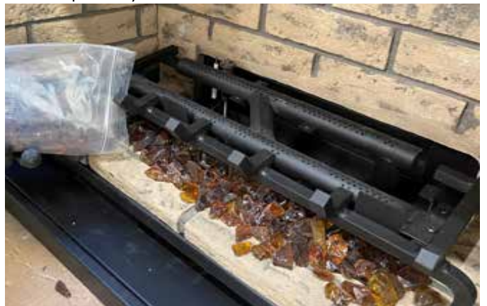
Diagram 3-Install Glass
