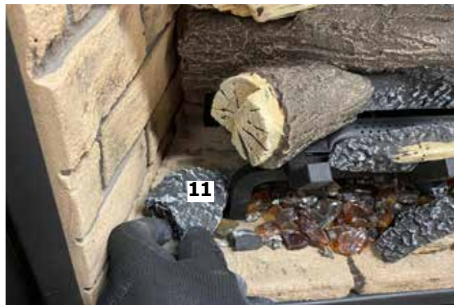
Diagram 16-Install Log 11
