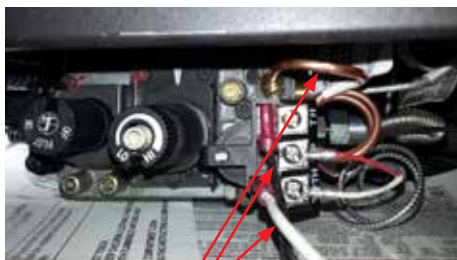
Diagram 4 Switch wires
