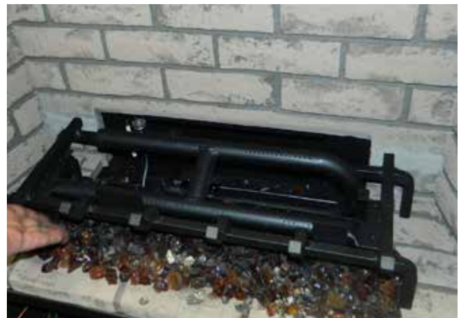
Diagram 4—Install Vermiculite + Lava
