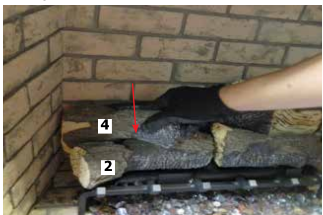
Diagram 10—Install Log 4
