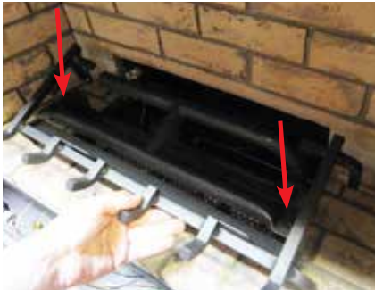
Diagram 1: Remove the left and right screws.
