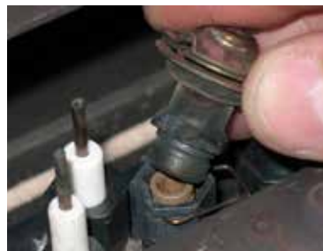
Diagram 2: Slide burner assembly to the right—then remove.
