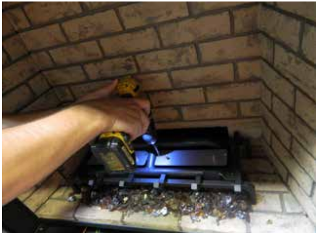
Diagram 5—Install Log support plates
