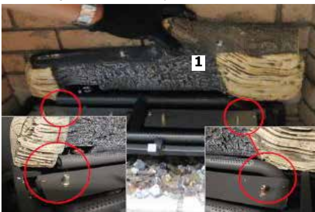
Diagram 7—Log 1 installation
