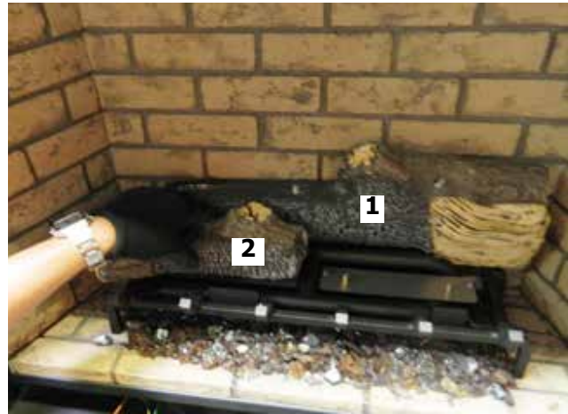
Diagram 8—Install Log 2
