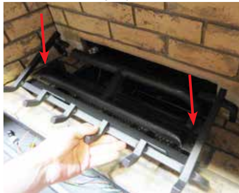
Diagram 1: Remove the left and right screws.
