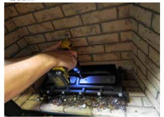
Diagram 5—Install Log support plates
