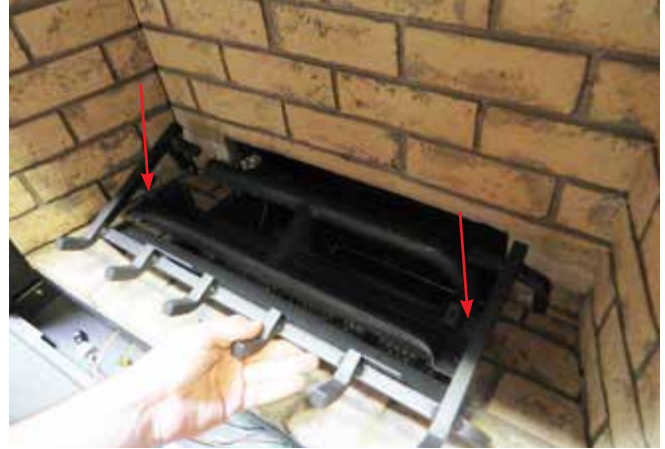
Diagram 2—Log Grate Install
