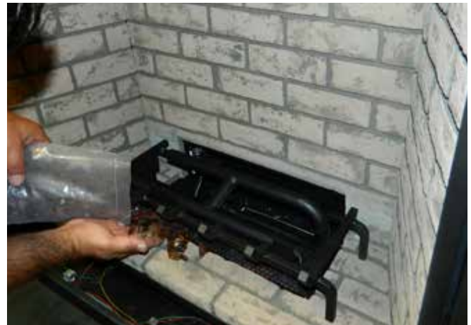
Diagram 3—Install Glass
