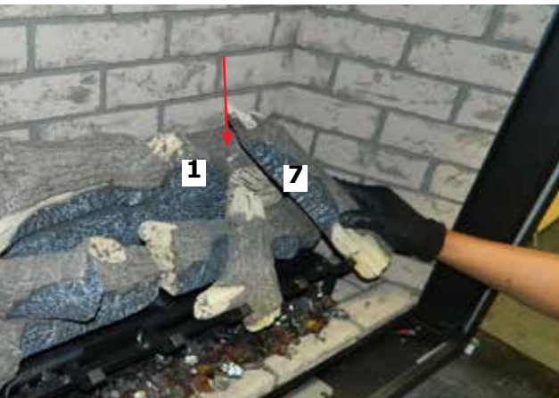
Diagram 13—Install Log 7
