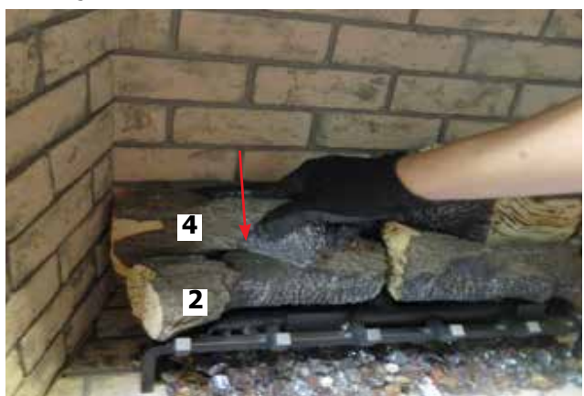
Diagram 10—Install Log 4
