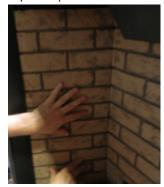
Slide the bottom panel carefully underneath the burner and push to the back until it contacts the back panel.
