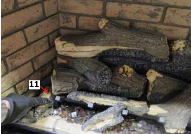
Diagram 17—Install Log 11
