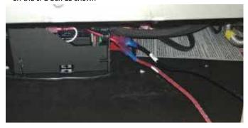
5. Connect fan ground cable to ground lug (located in lower right corner of unit). Refer to wiring diagram.
