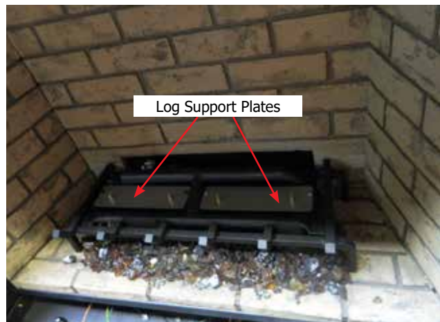
Diagram 6—Log support plates installed
