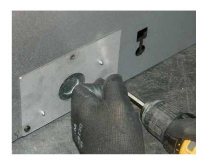
The electrical access panel is on the right side of the unit (when facing the front of unit).
