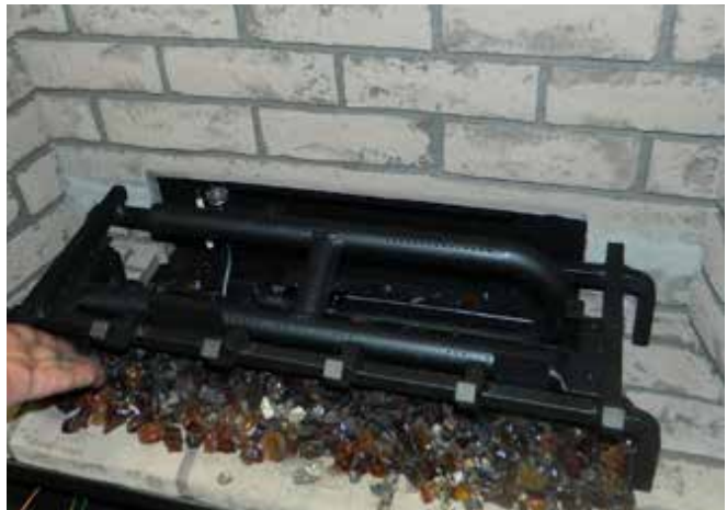
Diagram 4—Install Vermiculite + Lava
