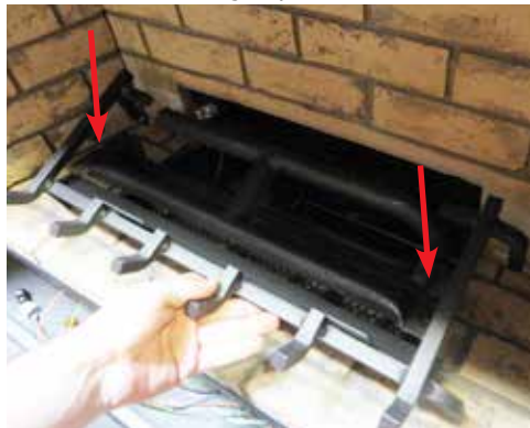
Diagram 1: Remove the left and right screws.
