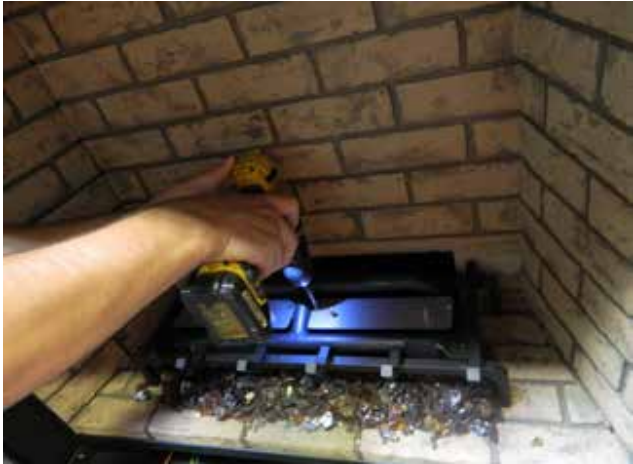
Diagram 5—Install Log support plates
