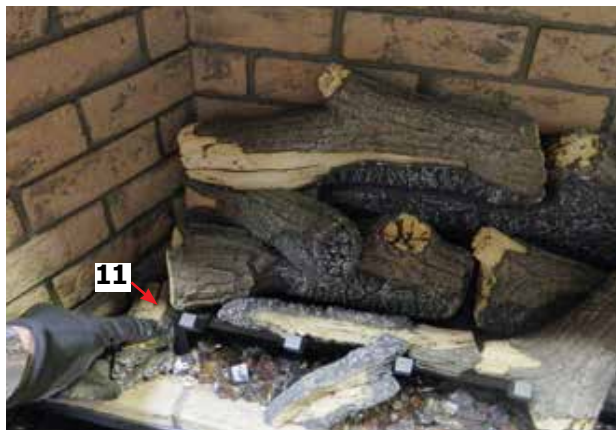
Diagram 17—Install Log 11
