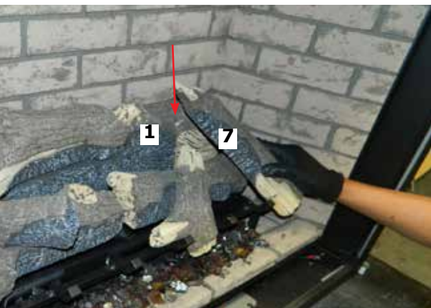
Diagram 13—Install Log 7
