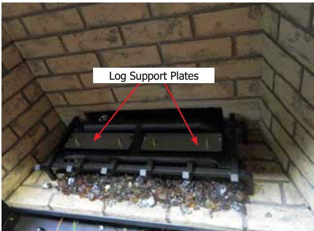
Diagram 6—Log support plates installed
