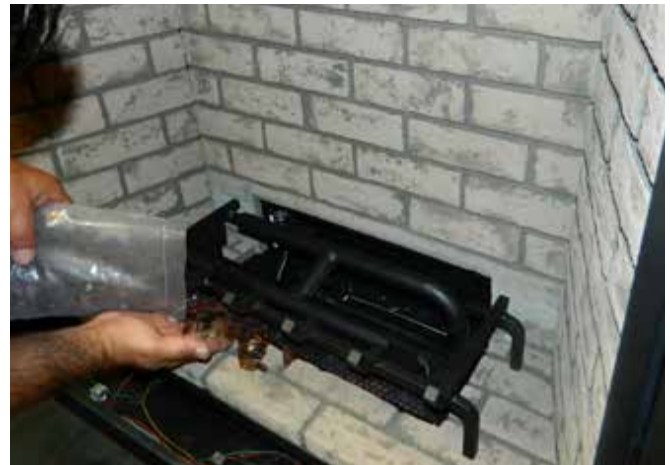
Diagram 3—Install Glass
