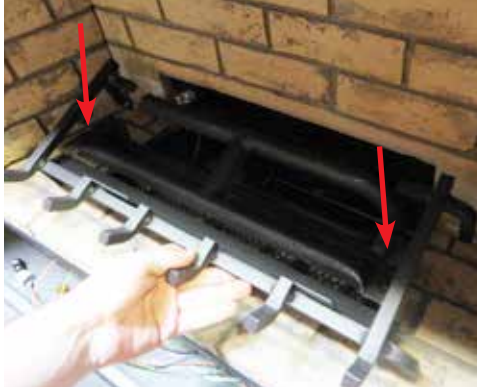
Diagram 1: Remove the left and right screws.
