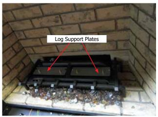
Diagram 6-Log support plates installed
