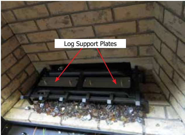
Diagram 6—Log support plates installed
