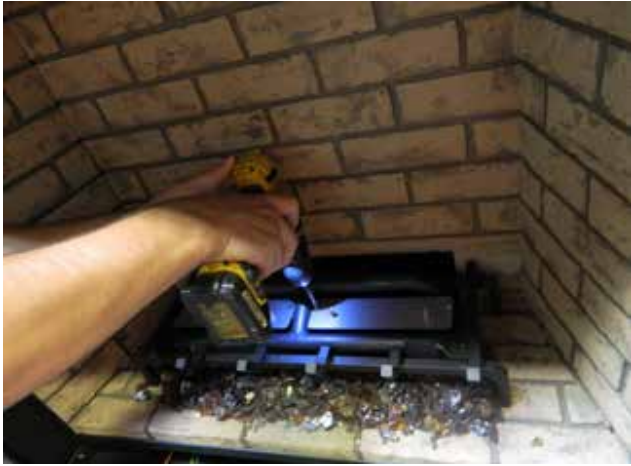
Diagram 5—Install Log support plates
