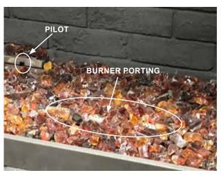
4. If using volcanic stones as additional media, add a maximum of 13, as shown below. Important: Volcanic stones should not cover any of the gas burner porting or pilot areas.
