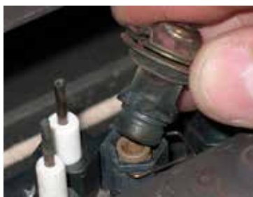
Diagram 2: Slide burner assembly to the right—then remove.
