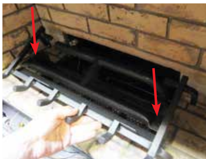
Diagram 1: Remove the left and right screws.
