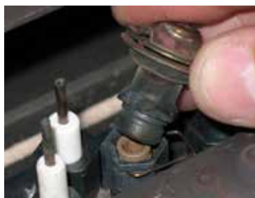
Diagram 2: Slide burner assembly to the right—then remove.
