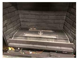
Attach the crystal tray with two screws, one on the middle left and another on the middle right of the tray, as shown below.
