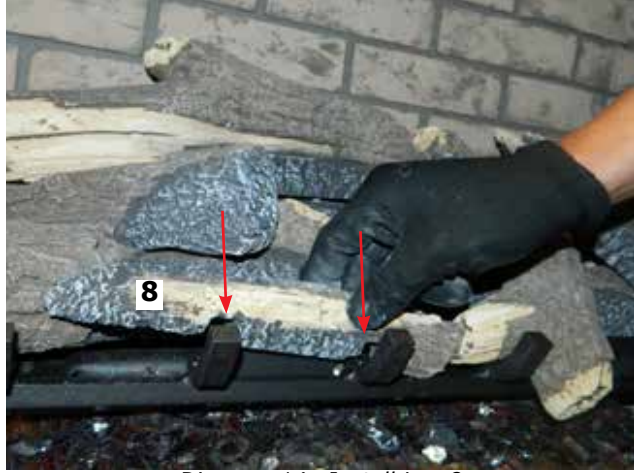
Diagram 14—Install Log 8
