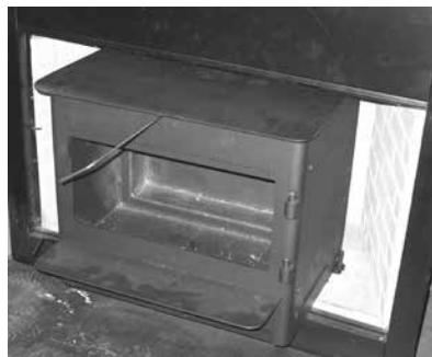
Pull Rod In Place
