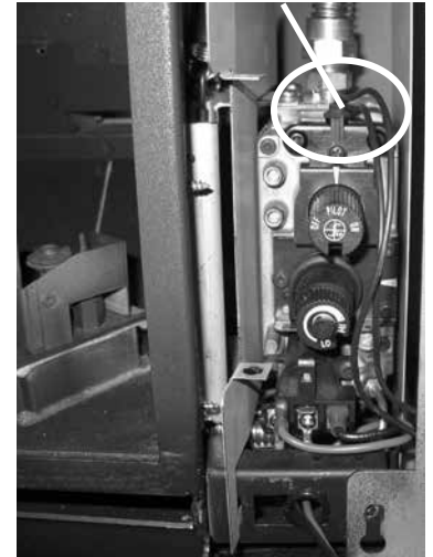
DC Sparker Wires
