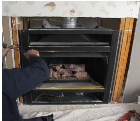
Remove unit from framing
