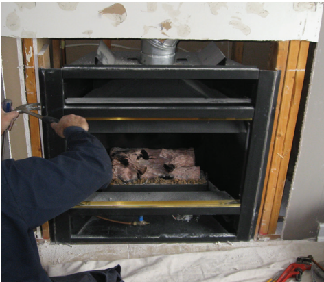
Remove unit from framing
