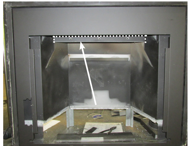
Cut out back cross bar
