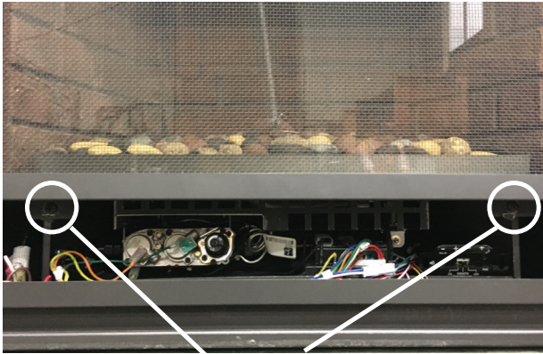
Retainer Screws Diagram 13.1
