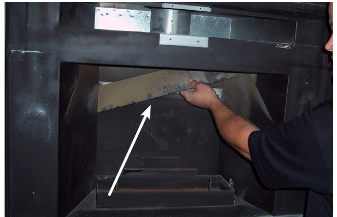
Remove rear baffle.
