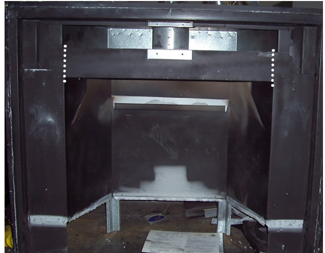
Cut out front cross piece to remove
