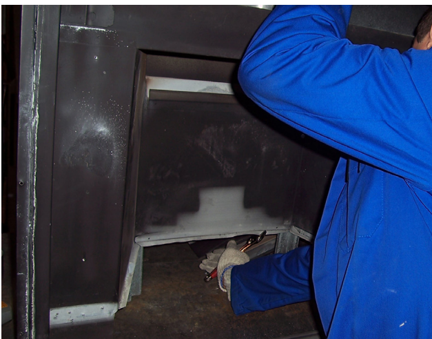
Flatten louver brackets
