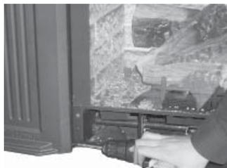
Install the glass trim by inserting the side hooks on the glass trim into the 4 slots between the faceplate and the glass. Push the glass trim down firmly with both hands to lock into place.
