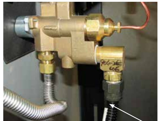
Diagram 11 Connect flex line to valve
