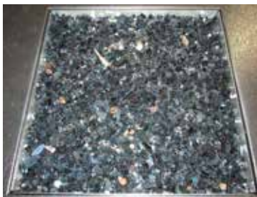
1. Spread crystals over burner. Base and burner tube should not be visible when complete. Do not cover thermocouple.
