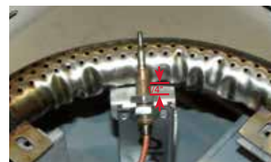
Diagram 4 - correct thermocouple position
