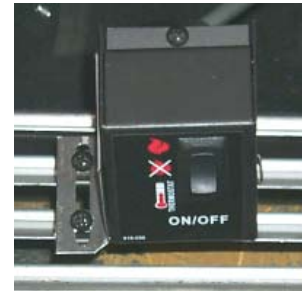
Burner ON/OFF control box attached to bottom flush louver.
