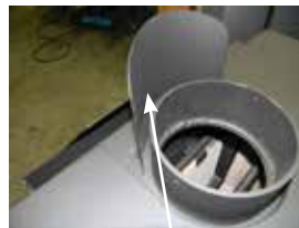
Installed Pipe Shield
