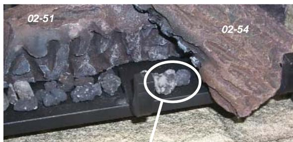
Do not block the burner ports in this area adjacent to the Log 02-54
