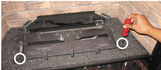
Diagram 1: Remove the left and right screws.
