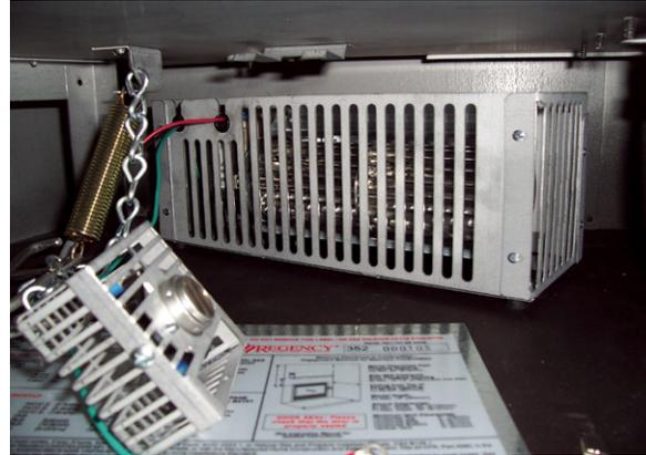
**NOTE:** If optional accent lights are installed, take care when sliding the fan into position. Fan must be maneuvered around the right side of the light.
