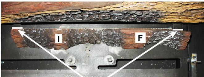
Diagram 5- location of back tabs on Burner
