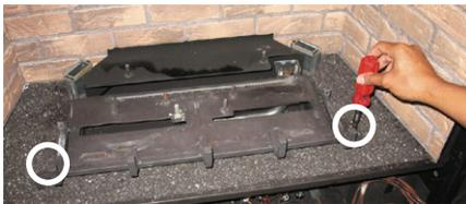
Diagram 1: Remove the left and right screws.
