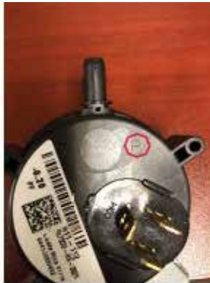
Pressure switch side "P"
